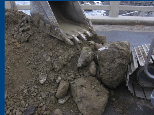
Approach fill between foundation abutments
