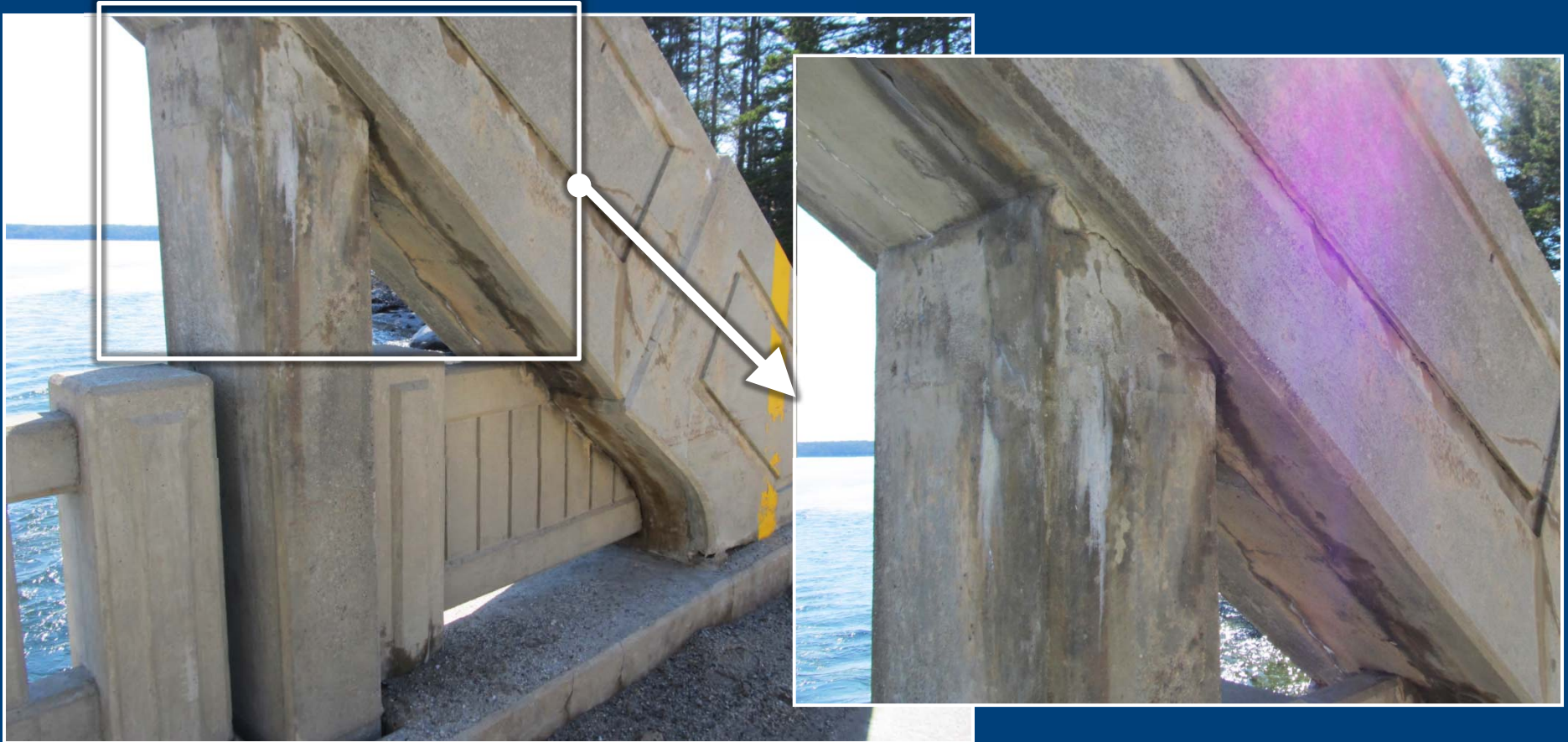
Deteriorating Concrete at Northwest Knuckle
