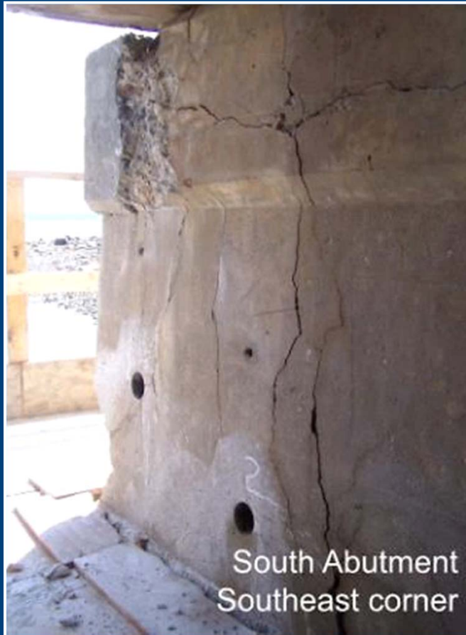
Concrete Spalling at Abutment
