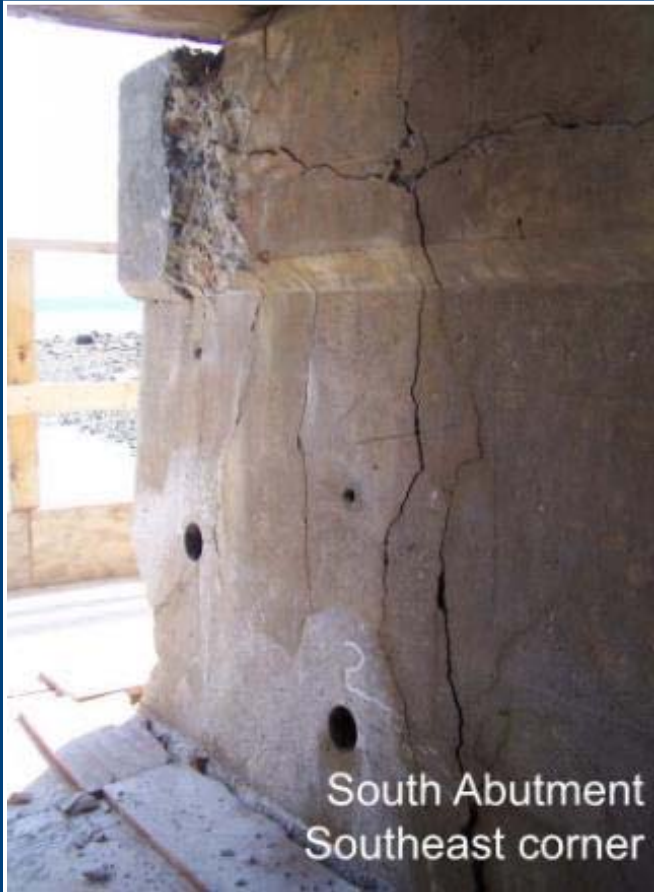
Concrete Spalling at Abutment
