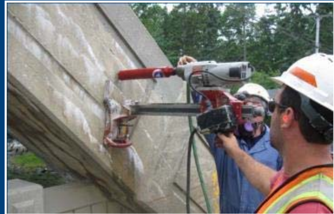
Concrete Coring
