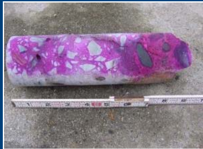
Concrete Core w/ Dye Penetrant
