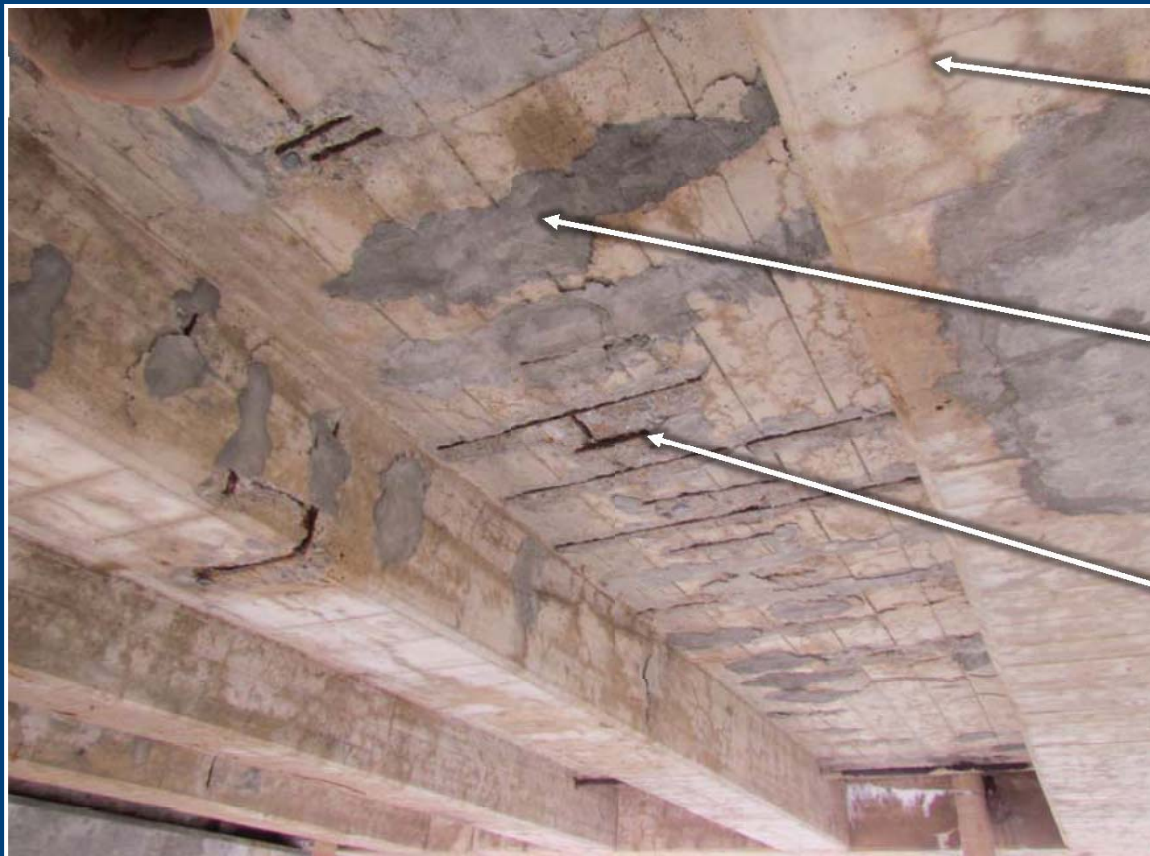
Deterioration on Underside of Deck
