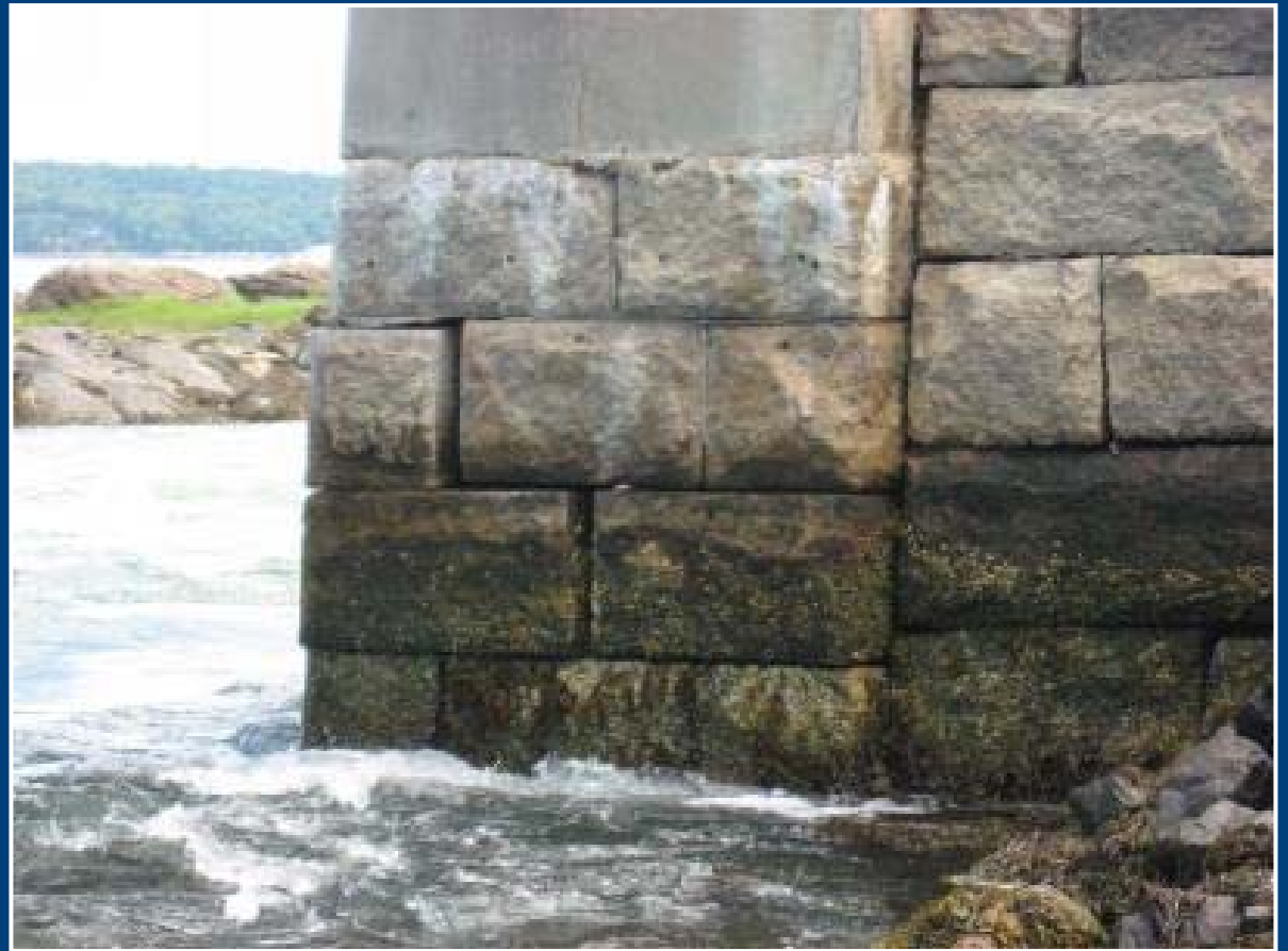
Settling Masonry
