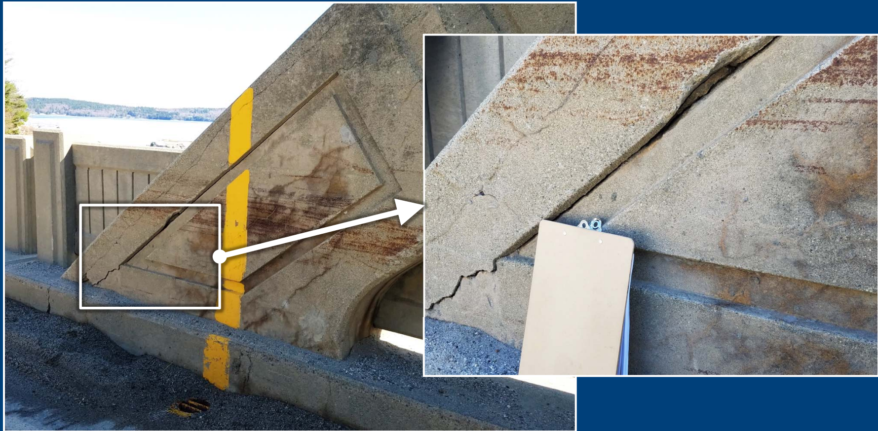
Deteriorating Concrete at Northeast Knuckle
