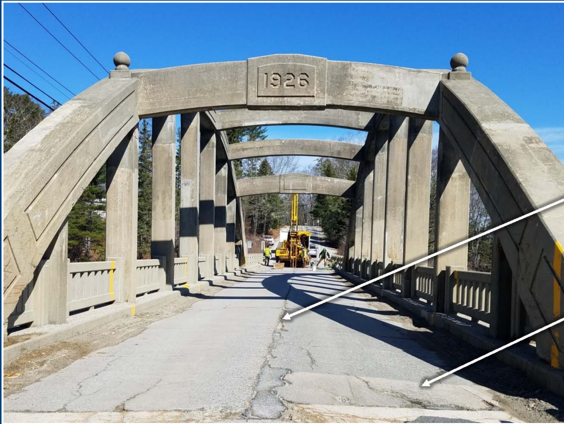
Deterioration at Deck Roadway Level
