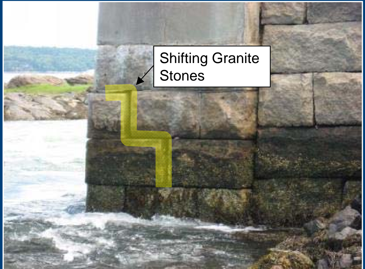
Settling & Shifting Masonry
