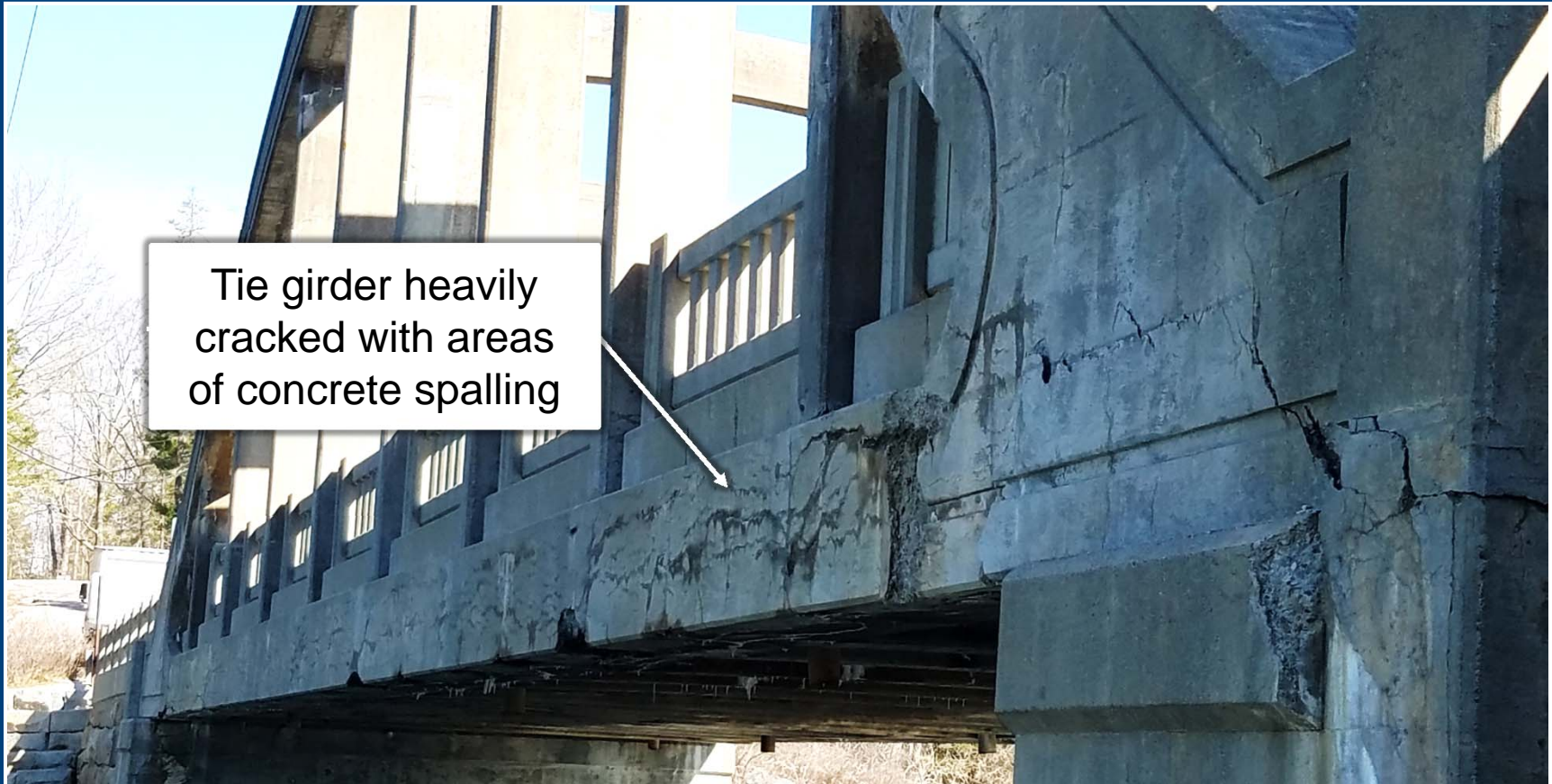
West Arch Tie Girder
