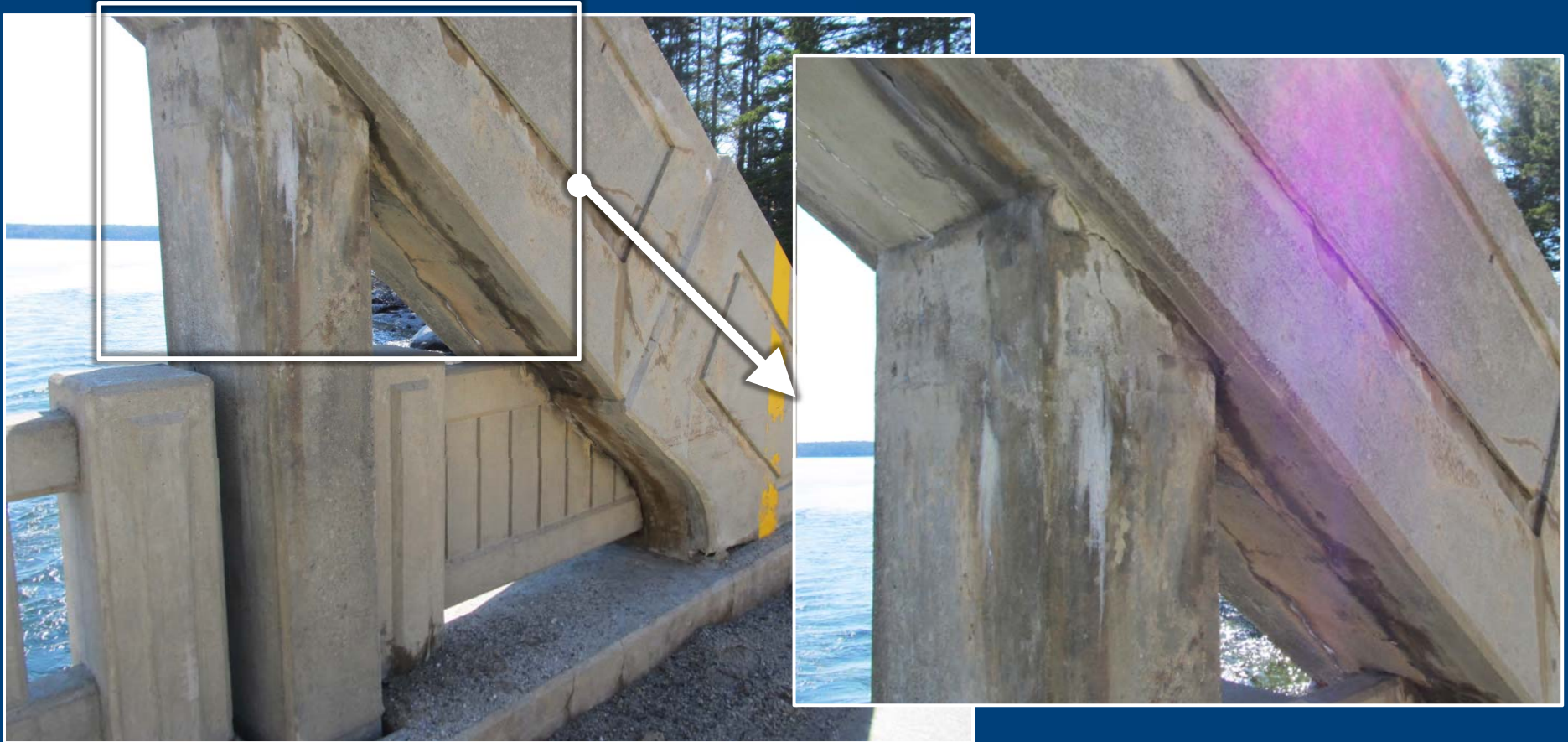
Deteriorating Concrete at Northwest Knuckle
