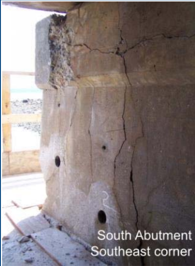
Concrete Spalling at Abutment
