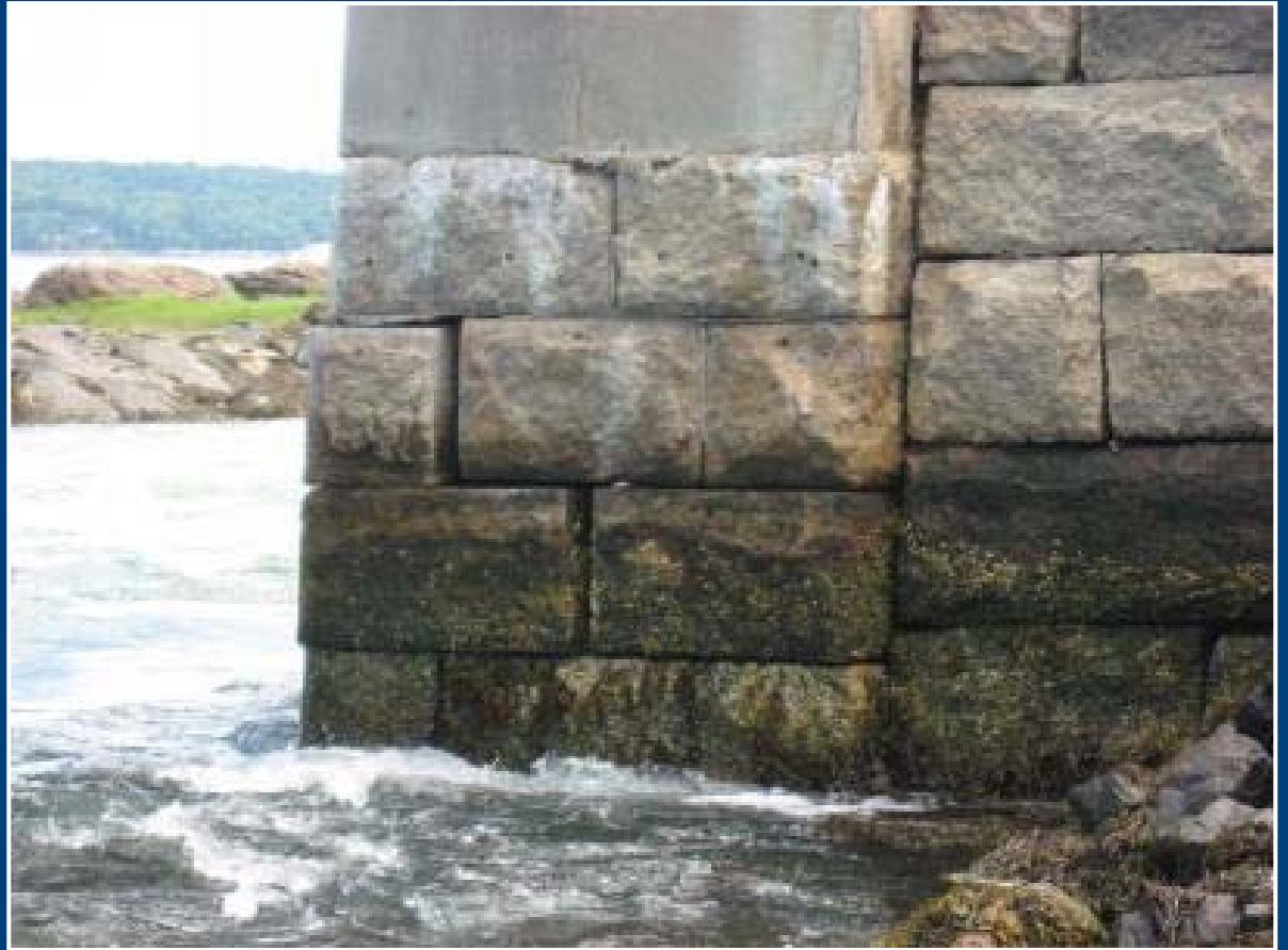
Settling Masonry
