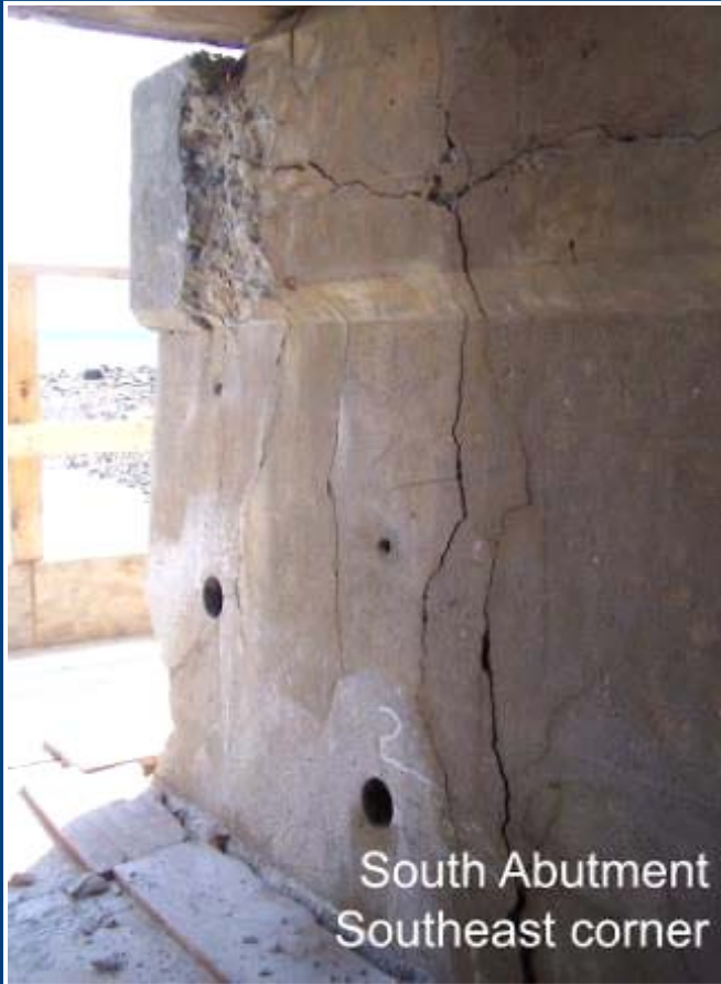
Concrete Spalling at Abutment
