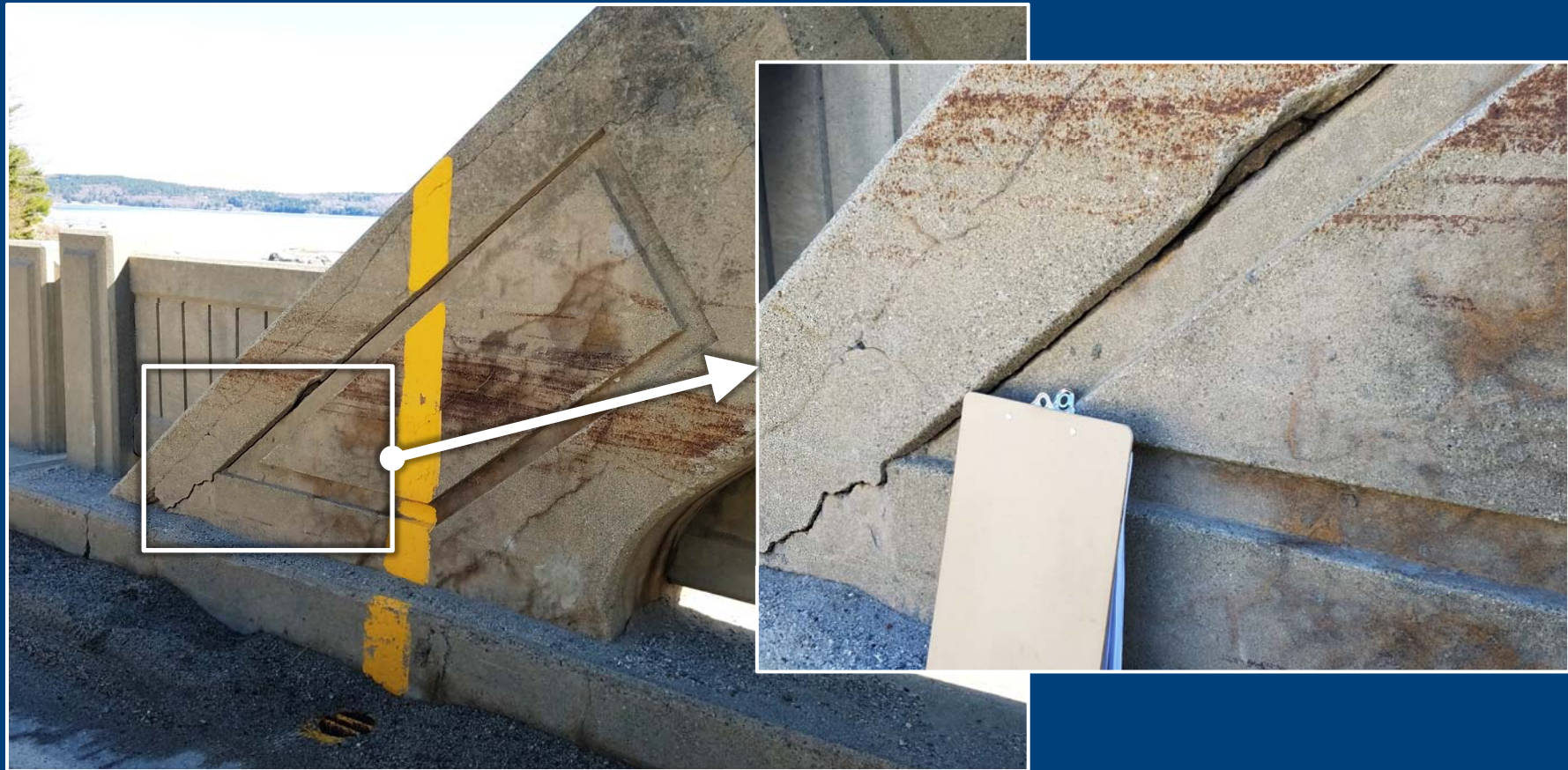
Deteriorating Concrete at Northeast Knuckle
