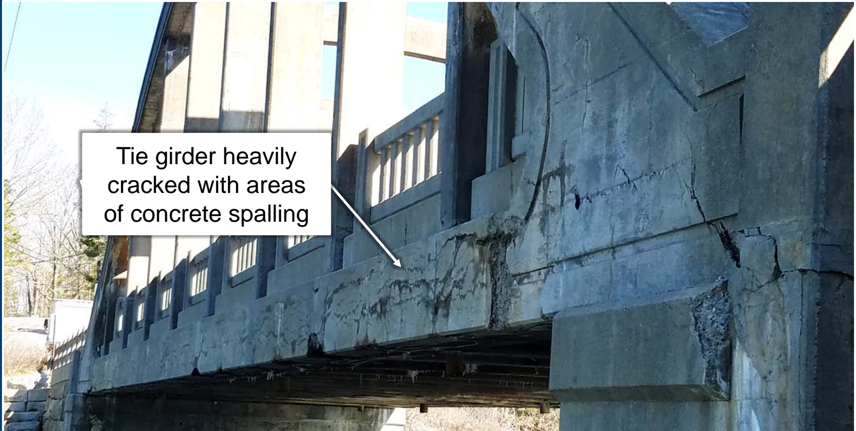
West Arch Tie Girder
