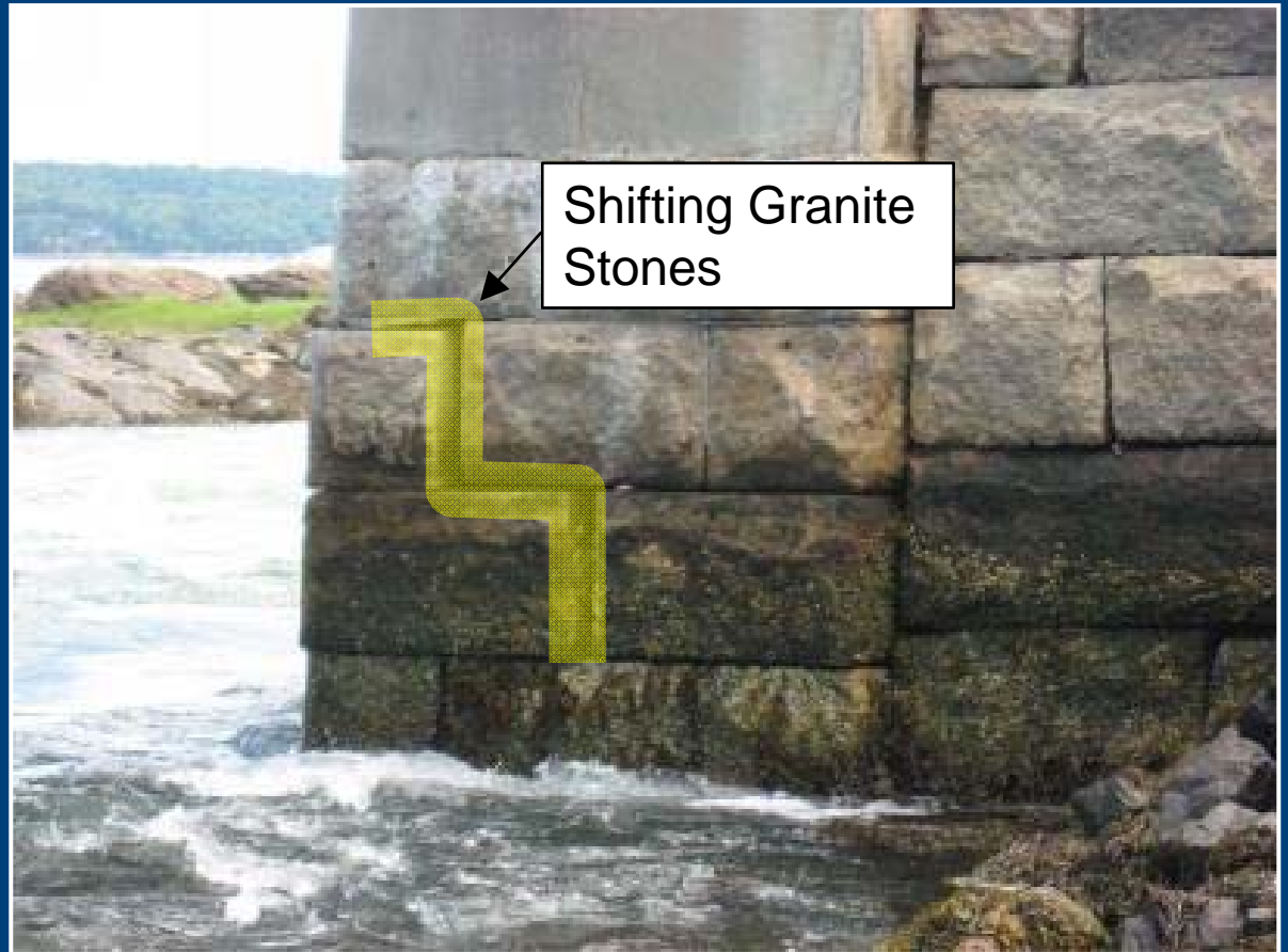
Settling & Shifting Masonry
