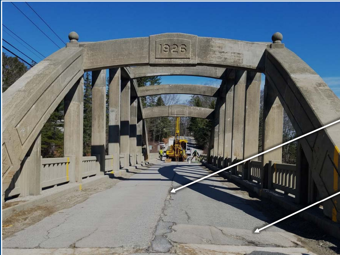
Deterioration at Deck Roadway Level
