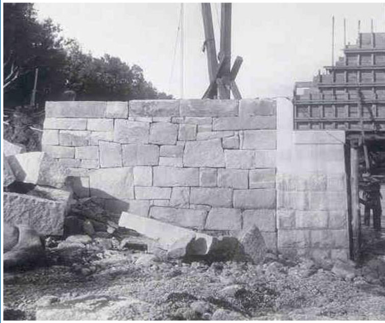
Wall During Construction (note voids are smaller and less frequent)
