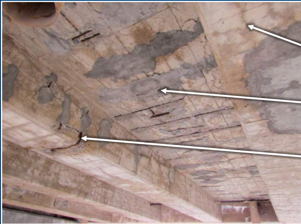
Deterioration on Underside of Deck
