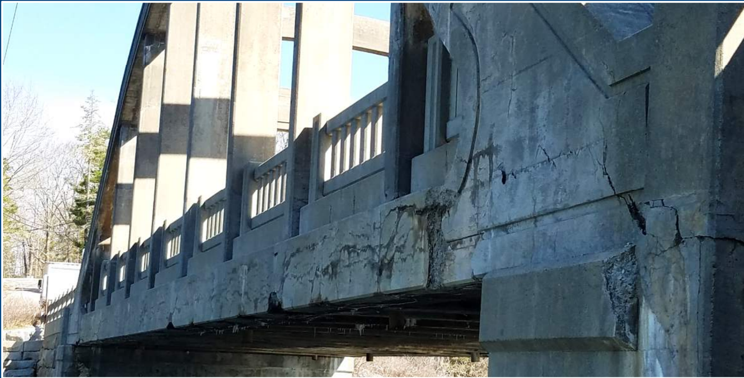
West Arch Tie Girder
