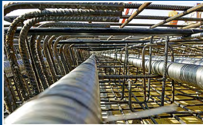
STRAND DUCTS INSTALLED
