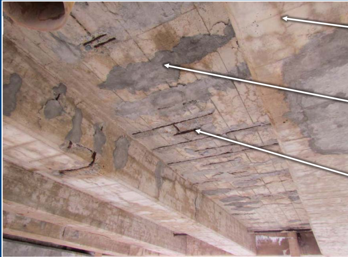
Deterioration on Underside of Deck
