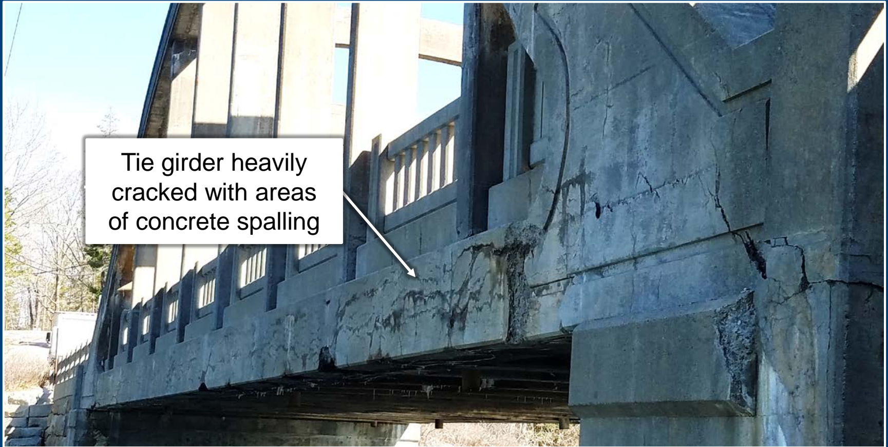
West Arch Tie Girder
