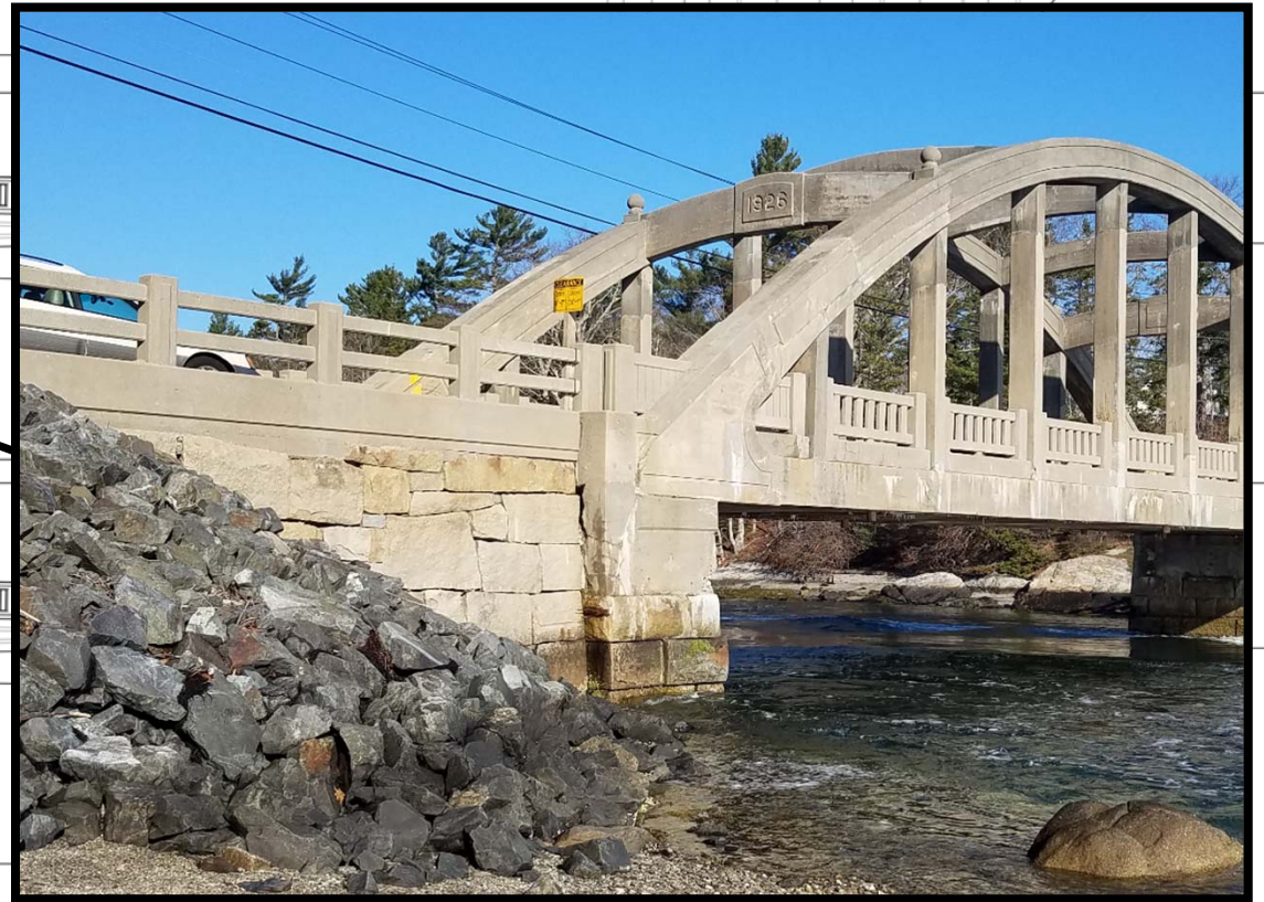
Existing Falls Bridge
