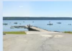
South Blue Hill Wharf
