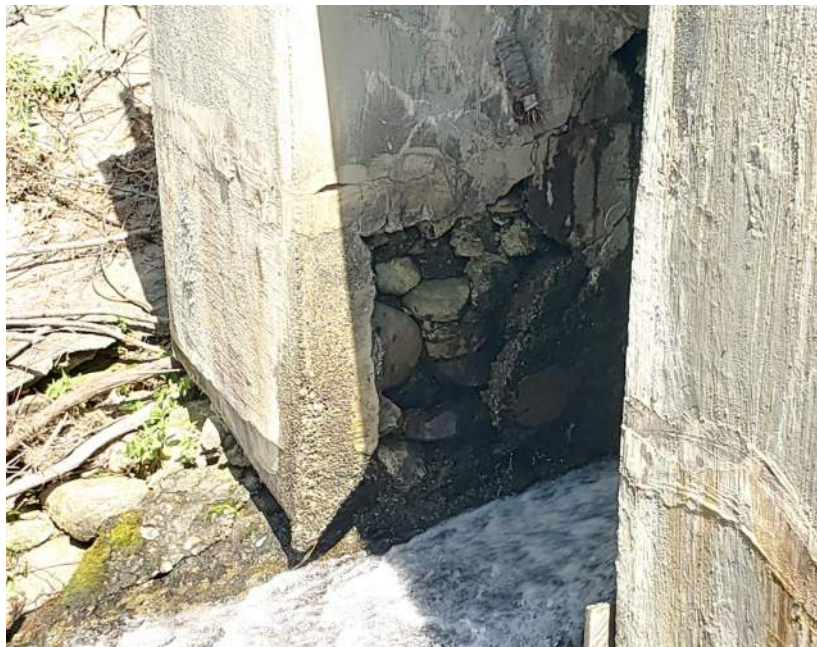
Photo No. 10 – Close up view of gate structure from the left embankment, looking right/upstream while the gate was opened. Note concrete loss.
