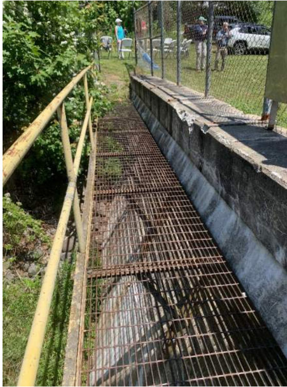
Photo No. 13 – View of access walkway, railing, and right abutment from the top of the intake structure, looking right. Note efflorescence and spalling.
