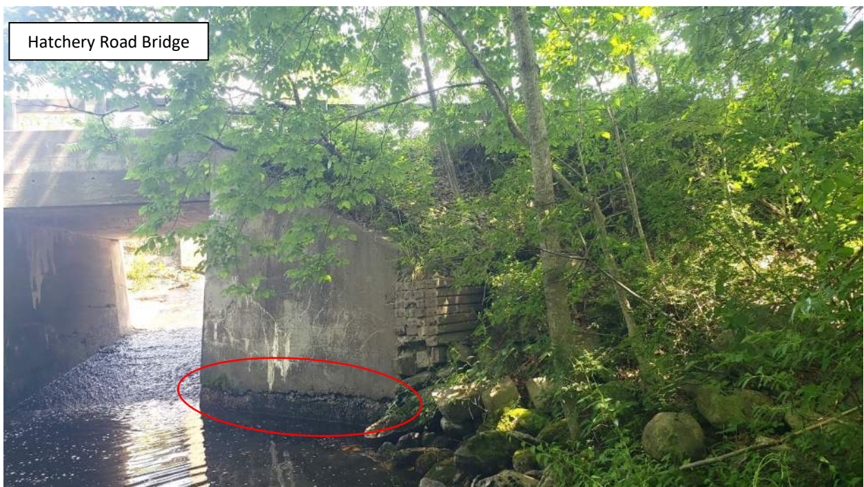
Photo No. 14 – View from left downstream shore, looking upstream toward the Hatchery Road bridge. Note concrete cracking and vegetation on the embankment.
