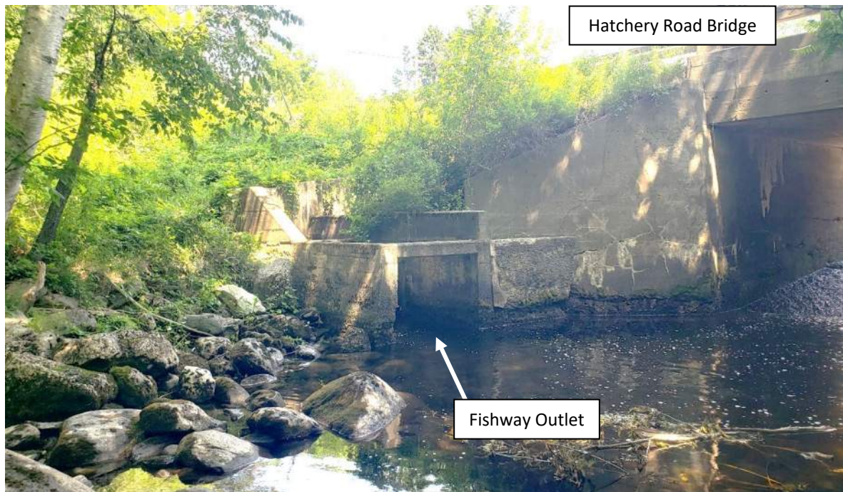
Photo No. 13 – View from left downstream shore, looking upstream toward the fishway outlet and Hatchery Road bridge. Note concrete loss and vegetation on the embankment.
