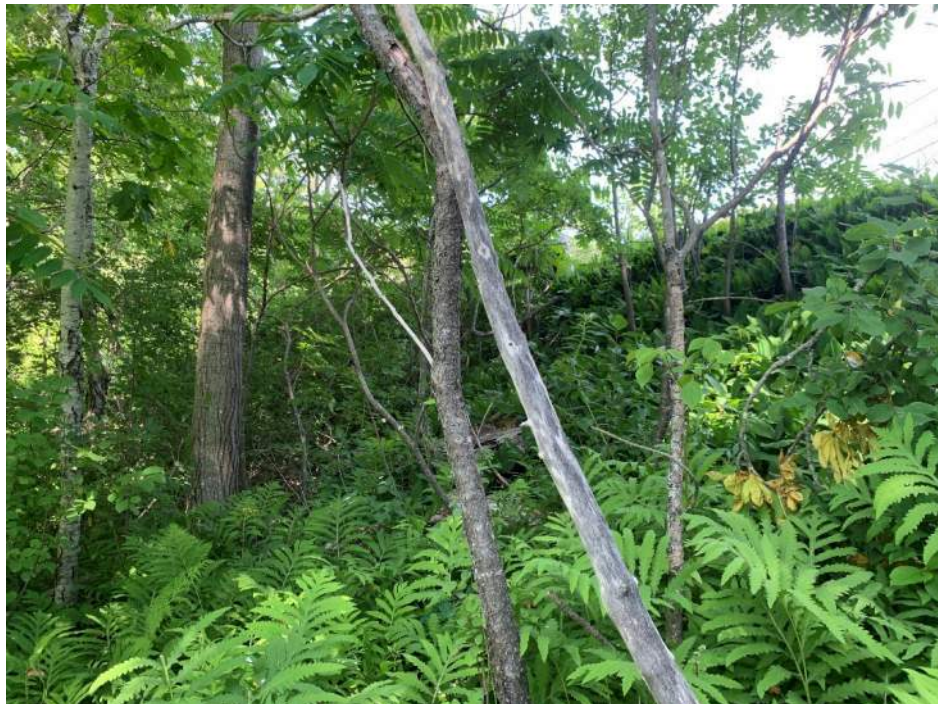
Photo No. 6 – Downstream side of left embankment (downstream of roadway), looking right. Note vegetation and large trees.
