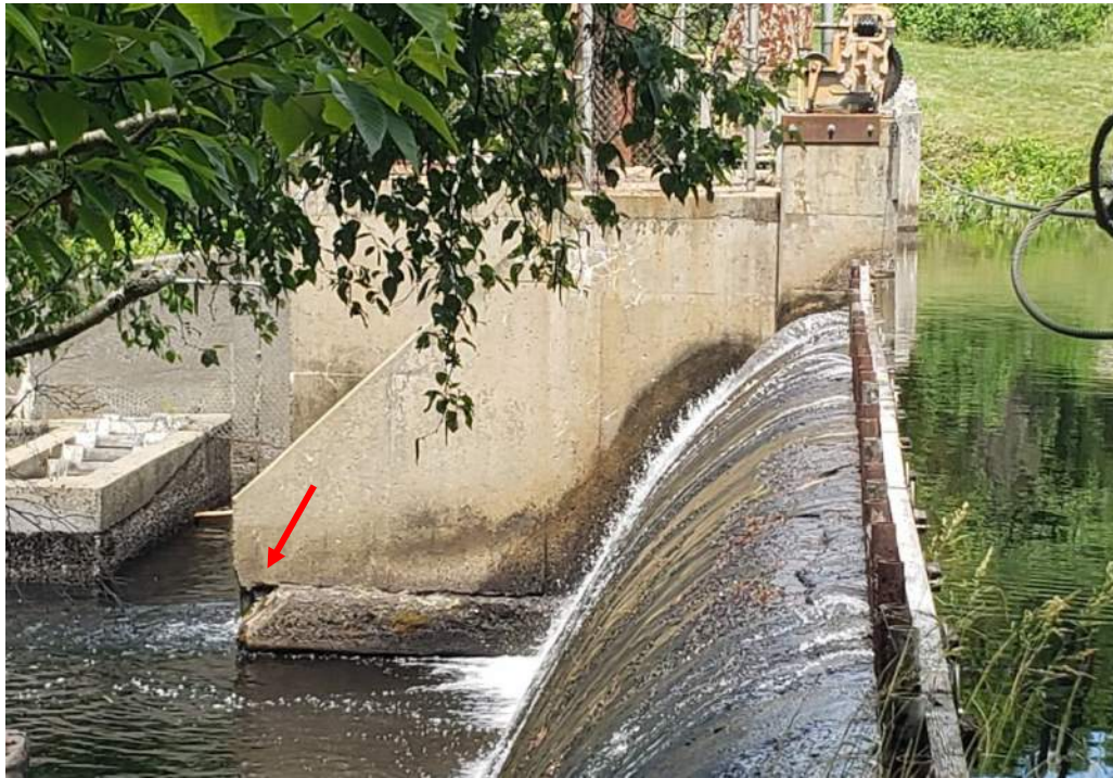
Photo No. 4 – View from left upstream shore, looking right. Note cracking and concrete loss on gate pier.
