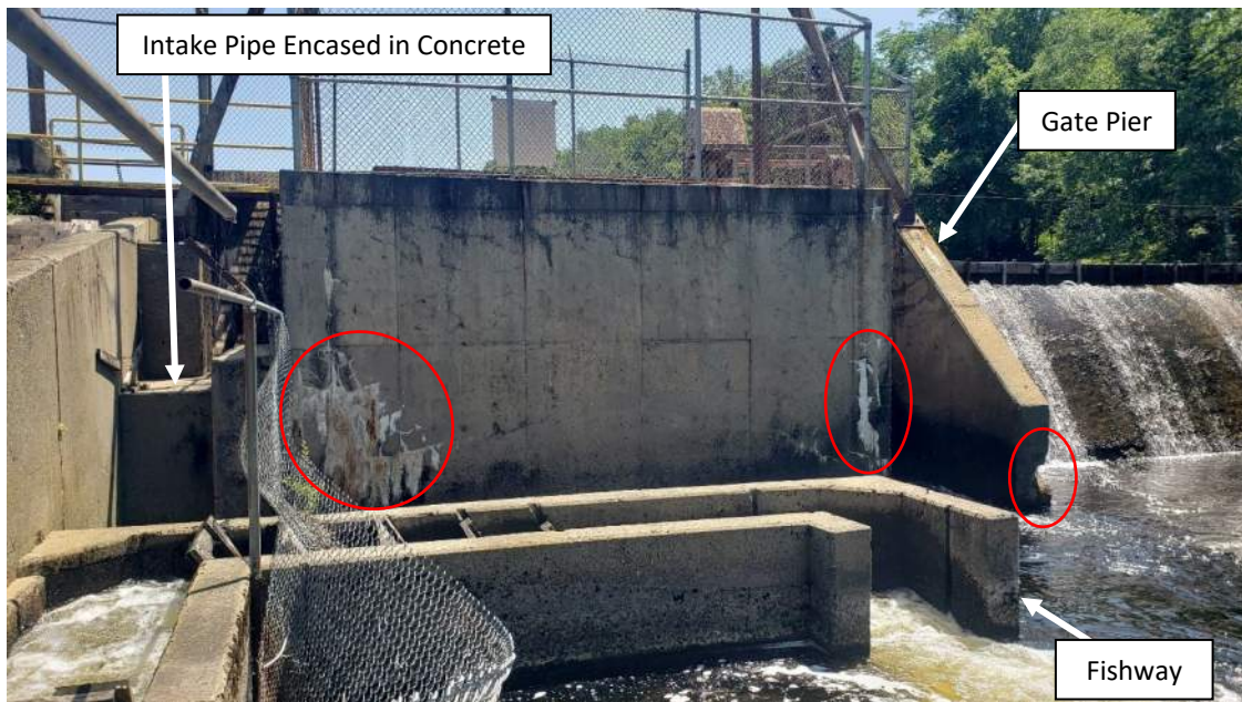
Photo No. 8 – View of fishway, intake structure, gate outlet, and spillway from right downstream shore, looking upstream. Note efflorescence on the intake structure, concrete loss on the gate pier, and the broken chain link fence.
