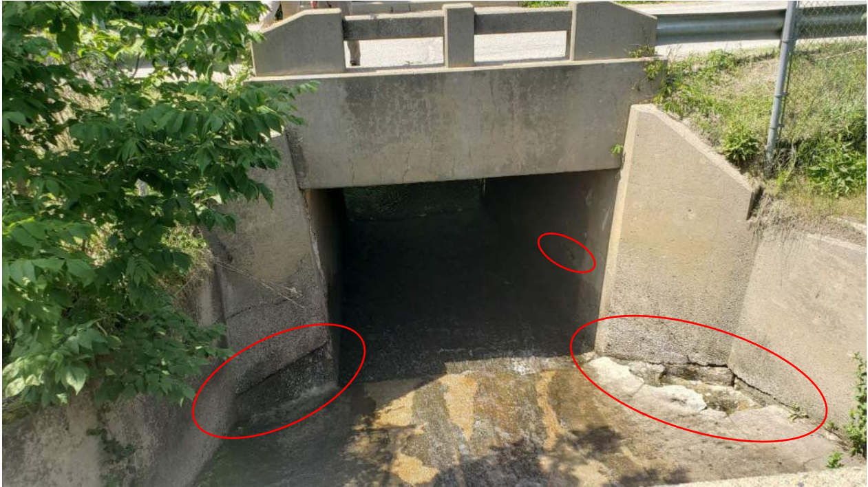
Photo No. 20 – View from top of gate looking downstream toward Hatchery Road bridge. Note cracking and concrete loss.
