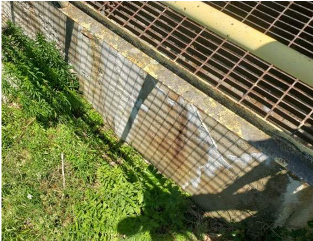
Photo No. 14 – View of the right abutment, looking down over the railing of the access walkway. Note efflorescence.
