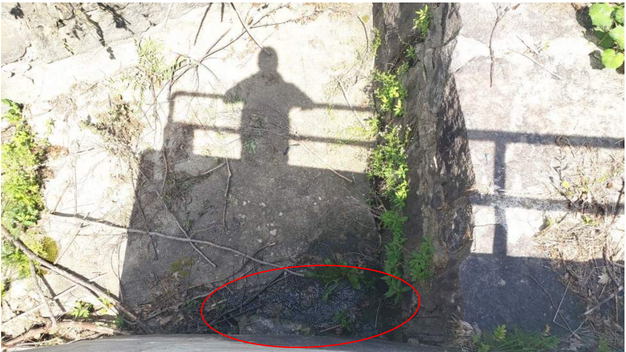
Photo No. 23 – View of right spillway and apron from top of gate, looking down. Note seepage.
