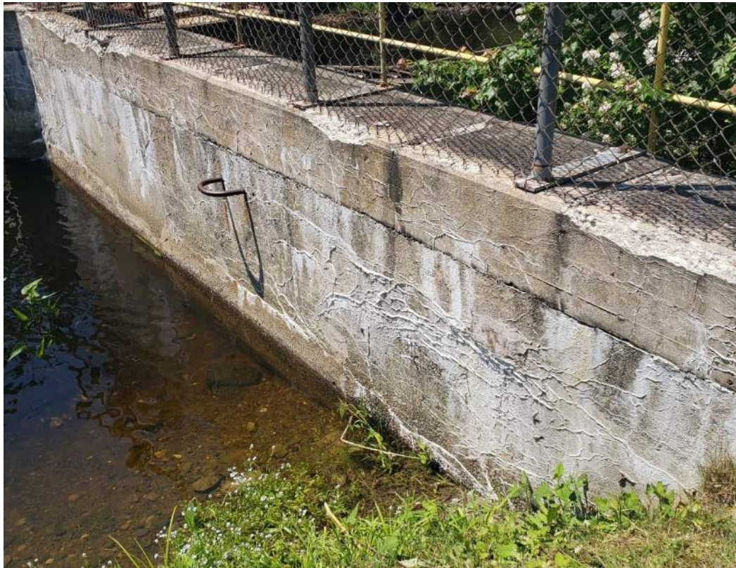
Photo No. 12 – View of right abutment from upstream right bank. Note efflorescence and spalling.
