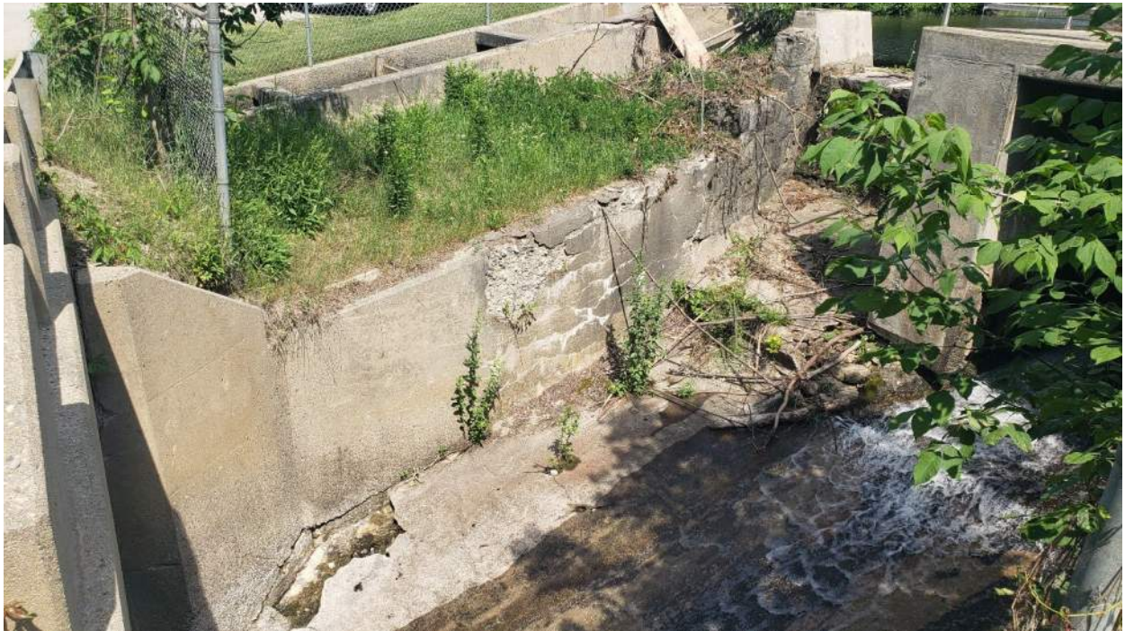
Photo No. 11 – View of dam from Hatchery Road bridge, looking upstream while the gate was opened. Note concrete loss on the right training wall and apron.
