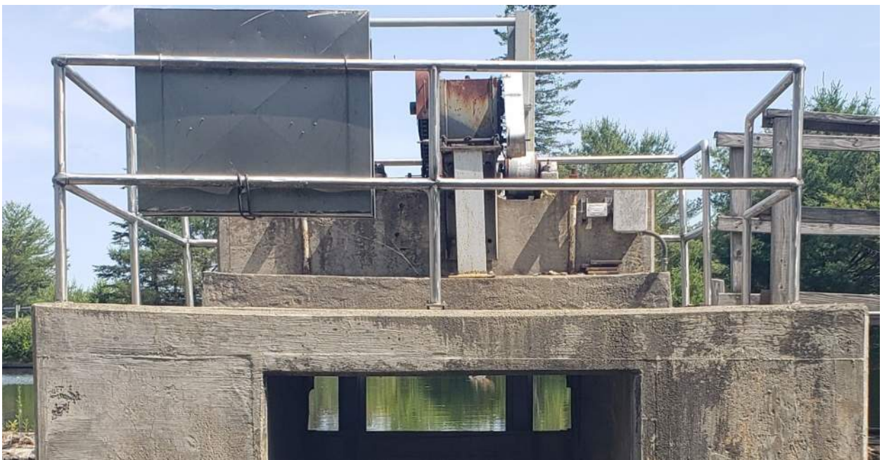
Photo No. 8 – View of the gate structure/operator platform from Hatchery Road bridge, looking upstream. Note the deflection of the concrete slab.
