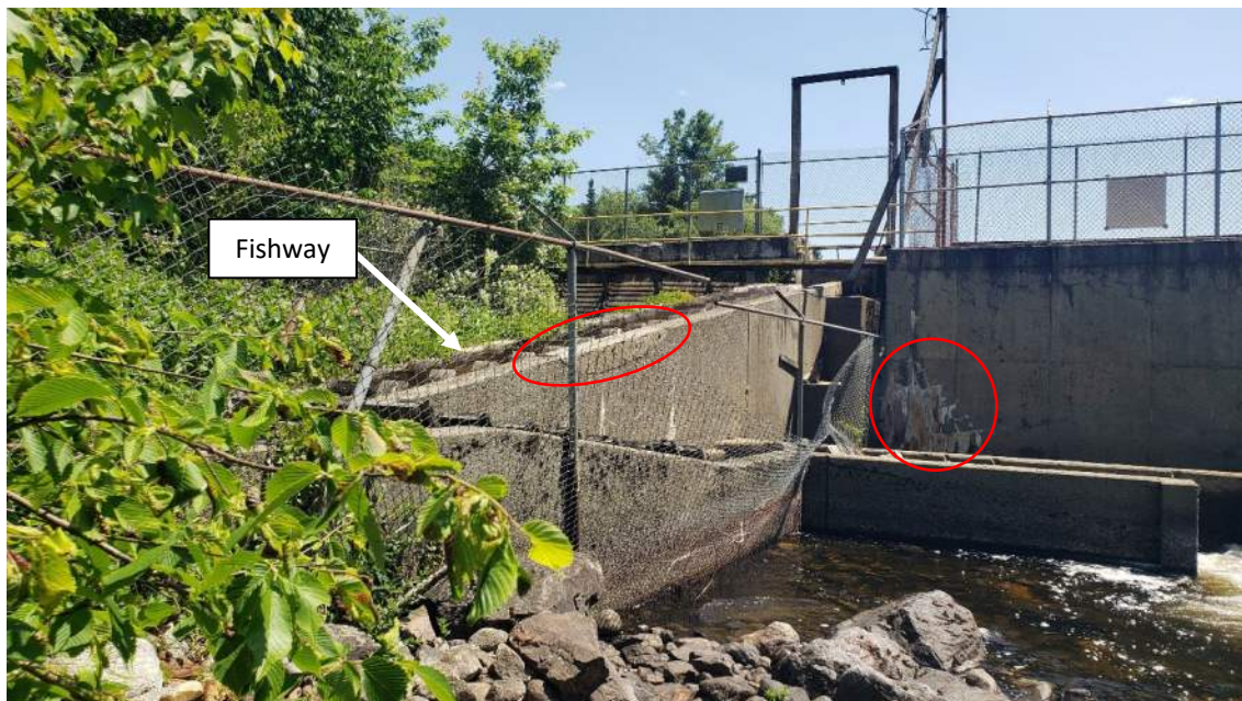
Photo No. 7 – View of fishway and intake structure from right downstream shore, looking upstream. Note efflorescence on the intake structure, repaired concrete on the fishway, and the broken chain link fence.
