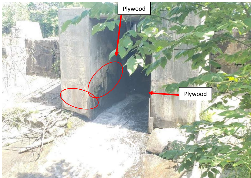
Photo No. 9 – View of dam from Hatchery Road bridge, looking upstream while the gate was opened. Note concrete loss. Plywood has been installed on the inside walls of the gate structure.
