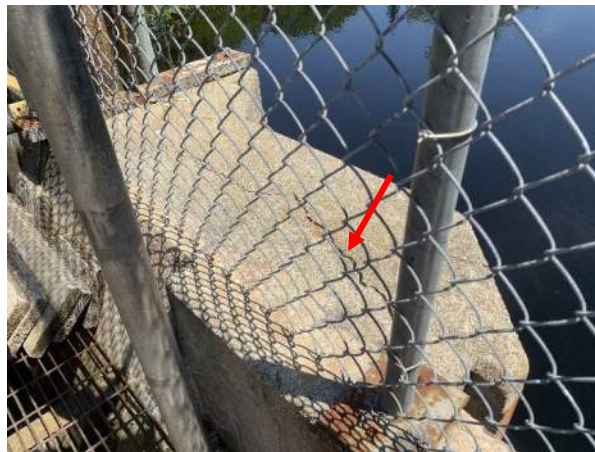
Photo No. 20 – View of concrete between fishway and intake structure from the top of the intake structure, looking upstream. Note cracking.
