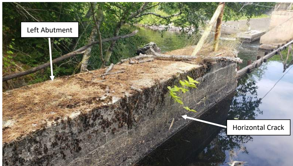
Photo No. 5 – View of left abutment from left upstream bank.
