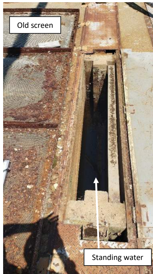
Photo No. 16 – View of open center hatch on top of intake structure, looking right. Old unused screen visible downstream of open hatch. Standing water was visible beneath the hatch.
