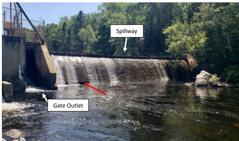
Photo No. 9 – View of gate outlet and spillway from right downstream shore, looking upstream. Note deterioration at concrete lift joint (red arrow).
